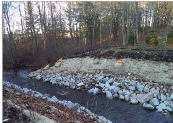
“After” photo of culvert removal site.
