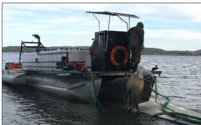
The Auburn Water District used $400,000 in CWSRF to help carry out an alum treatment of Lake Auburn. The goal was to reduce phosphorus concentrations and algae growth in the lake, which serves as a public drinking water supply for over 46,000 residents.
