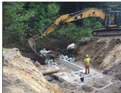
Installation of a Stream Smart crossing at River Road.
