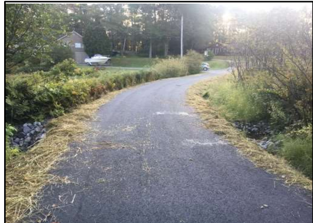
After: New, armored culvert and paved driveway
