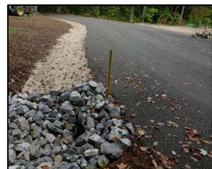
Pine Drive after BMPs installed
