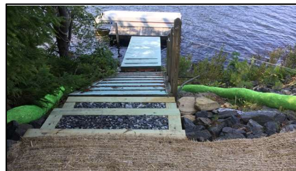
Infiltration steps installed at a property on Knickerbocker Lake.
