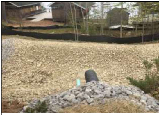
New 180' culvert and plunge pool installed to capture and filter runoff
