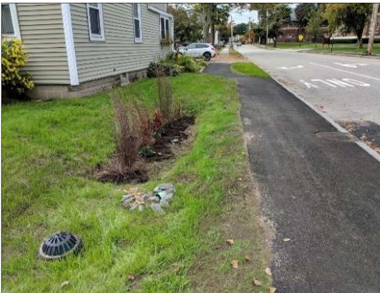
Stormwater retrofit project that featured a biofiltration system.
