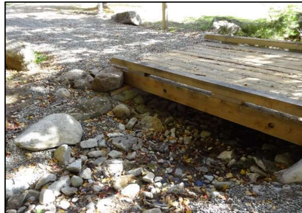
Bridge constructed to replace a failing culvert
